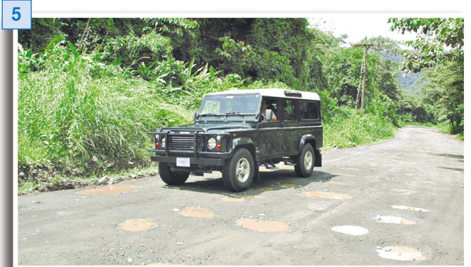
Poor road conditions
